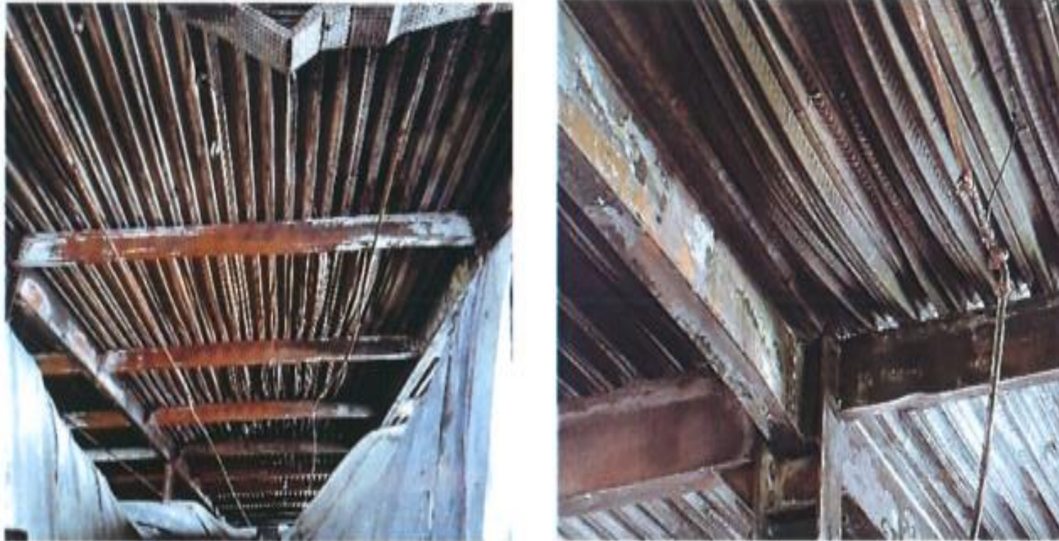
Figure 5.1- Damaged Steel deck and beam
