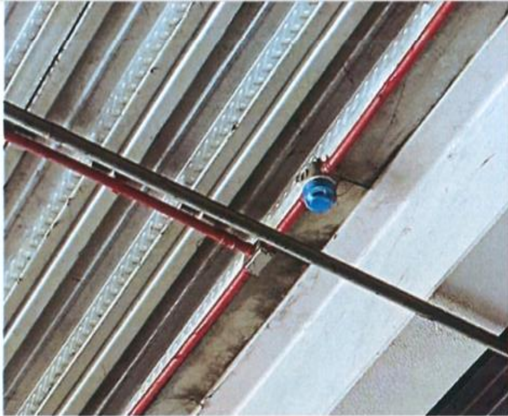
Figure 2.4 – Covered Smoke detectors
