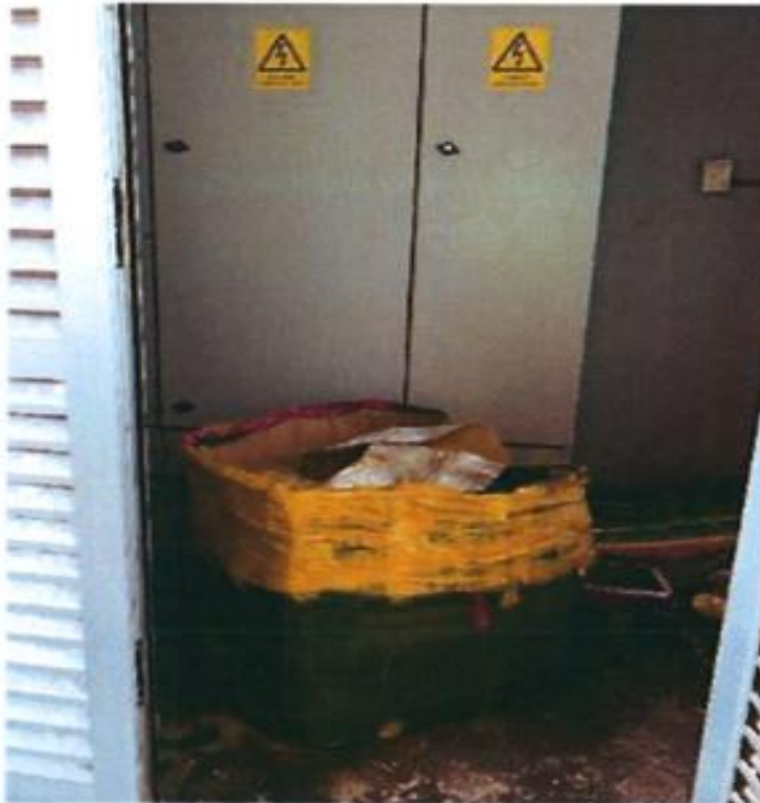
Figure 5.10- Electrical Room being used as storage
